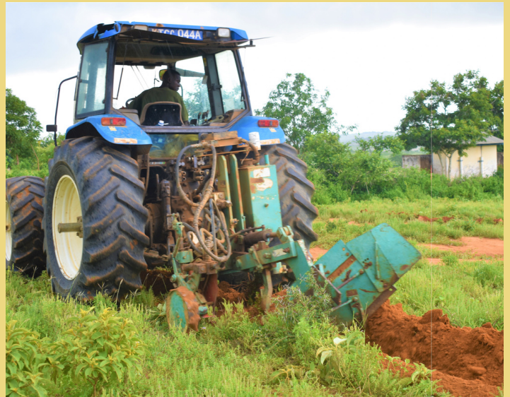
Ongoing construction of mechanized terraces at WRUAs
