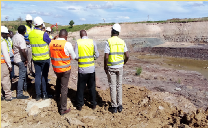
Monitoring progress at the on-going construction of the Mwache dam
