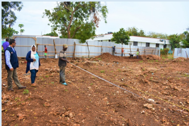
Ongoing construction of the ICU at the hospital
