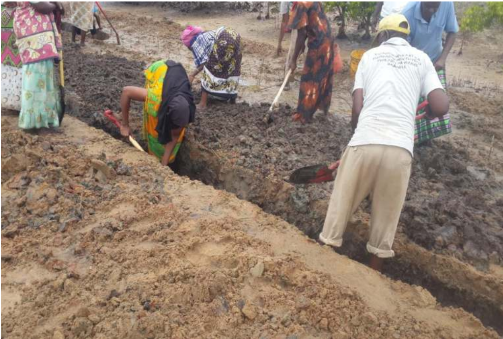
Site preparation at Jimbo in Vanga
