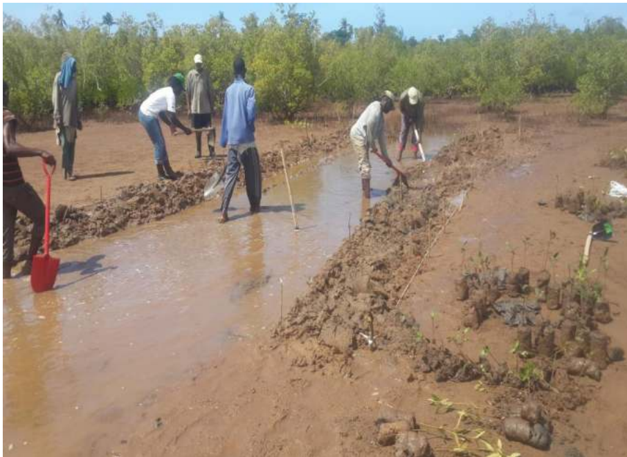
Preparing the Mwagugu site before planting
