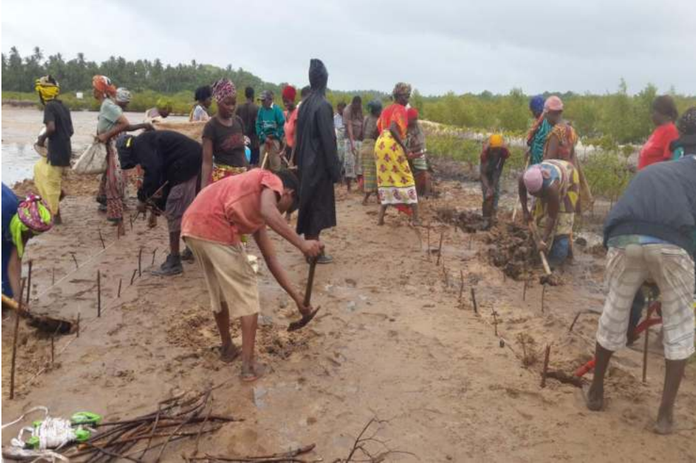
Site preparation at Makongeni Gazi
