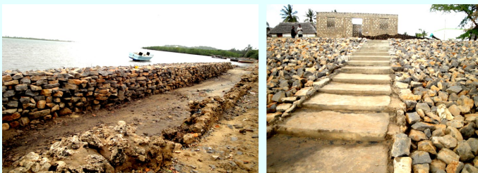
The Sea wall & its Stair case at Ngomeni village
