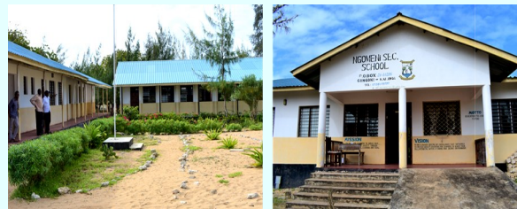
Construction of a new Ngomeni Secondary School
