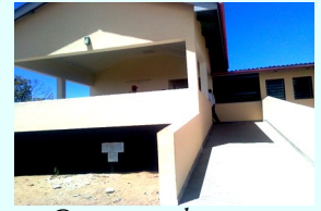
Constructed new Ngomeni Health Centre
